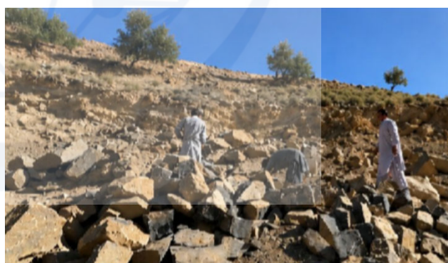
Figure 3 (a): Stone Collection and Selection - Locally sourced bluish is collected from nearby Outcrops and selected for Construction
