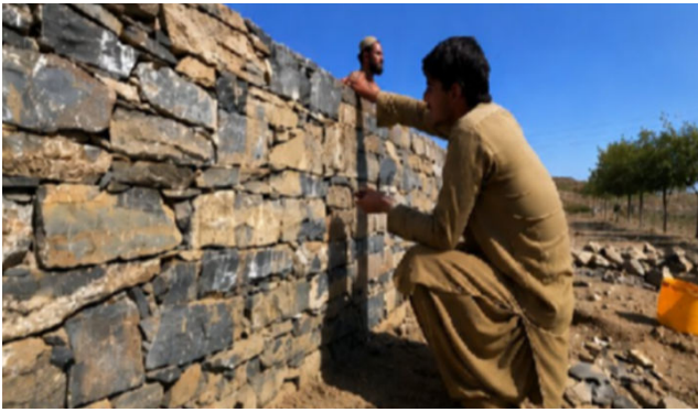
Figure 3 (b): Wall Construction Process – Stones are carefully placed one by one in proper alignment, ensuring Strength, Stability and Traditional craftsmanship
