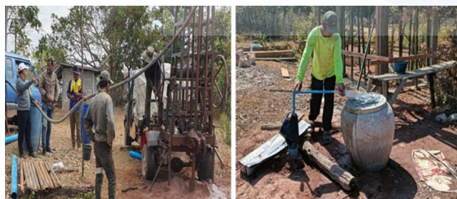
Figure 2: Groundwater Drilling and Water Quantity Test
