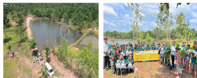
Figure 5: Public Village Pond Completed Construction and Fish Released
