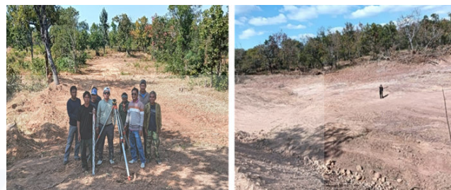
Figure 3: Public pond Infrastructure and Site Preparation
